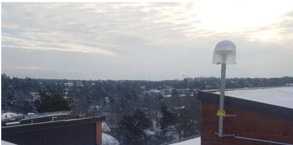
Figure 1.4: Gustavsberg is a SWEPOS class B station with a roof-mounted GNSS antenna mainly established for network RTK purposes.
