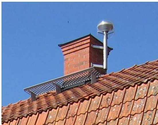
Figure 1.4: The SWEPOS station Söderboda, monumented on top of a building.
