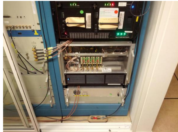
Figure 2.1: The new rack for VLBI at Onsala Space Observatory is a modern digital backend system.
