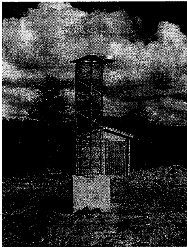
Fig. 2. Joensuu permanent GPS station Lat 62°23 Lon 30°06'. In the background is a small warmed cabin for the receiver.
