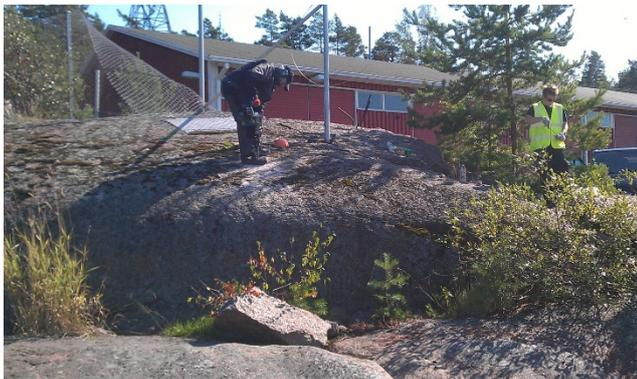
**Fig. 4.** Installation of a new benchmark near Porvoo tide gauge. Photo: V. Saaranen.
