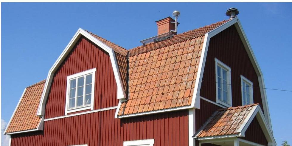
Figure 1.4: Söderboda is a SWEPOS station with a roof-mounted GNSS antenna mainly established for network RTK purposes belonging to class B.
